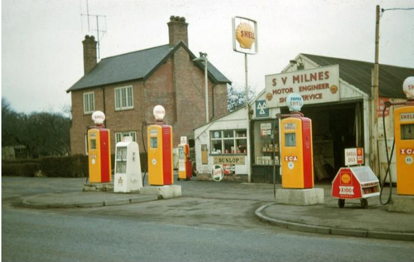
Milnes' garage on the Great North Road
