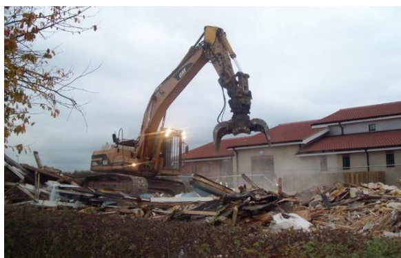
Demolition of the old village hall
