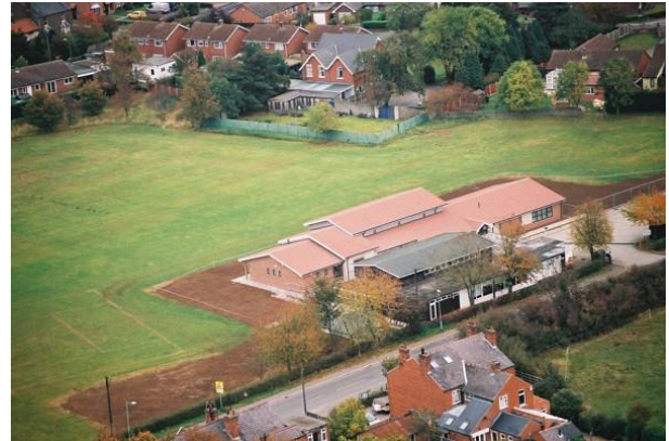
Aerial View of the new MRCC alongside the old Village Hall
