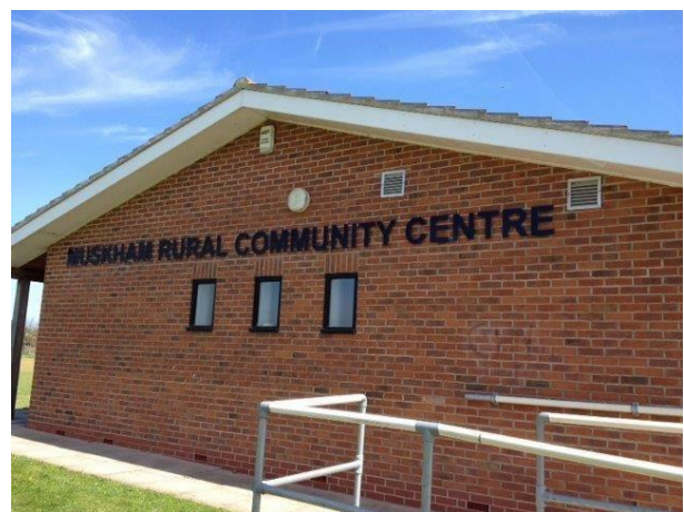
Changing room end of MRCC
